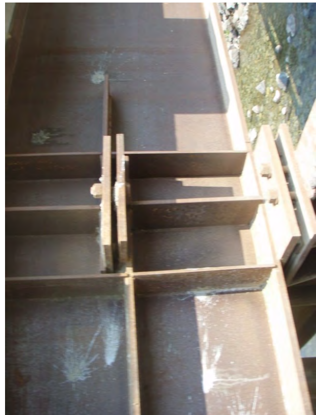
Figure 31: Span 2 bearing at Pier 1
