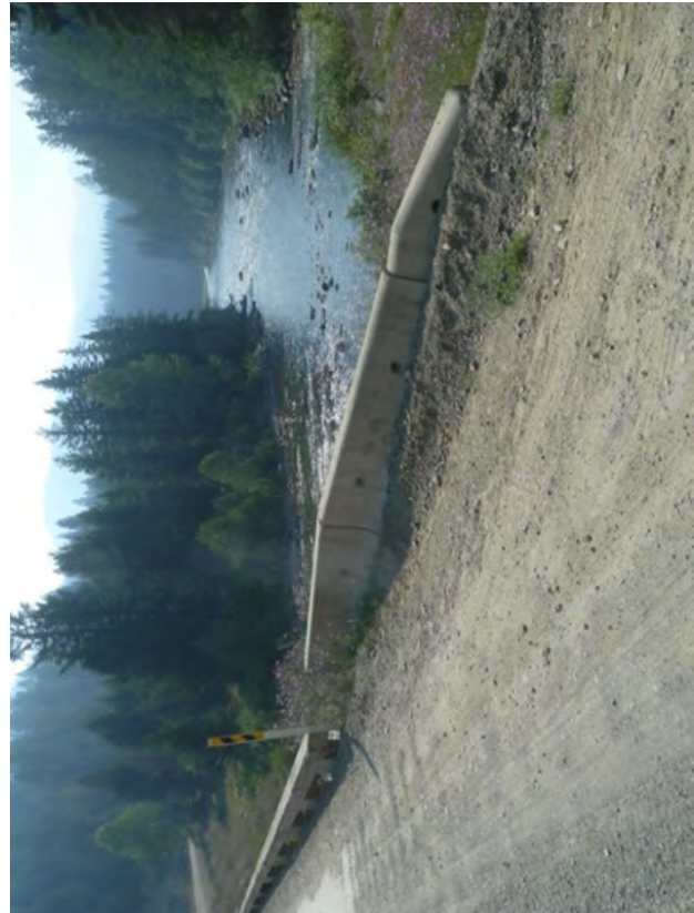
Figure 8: Typical approach flare - left upstream side shown.
