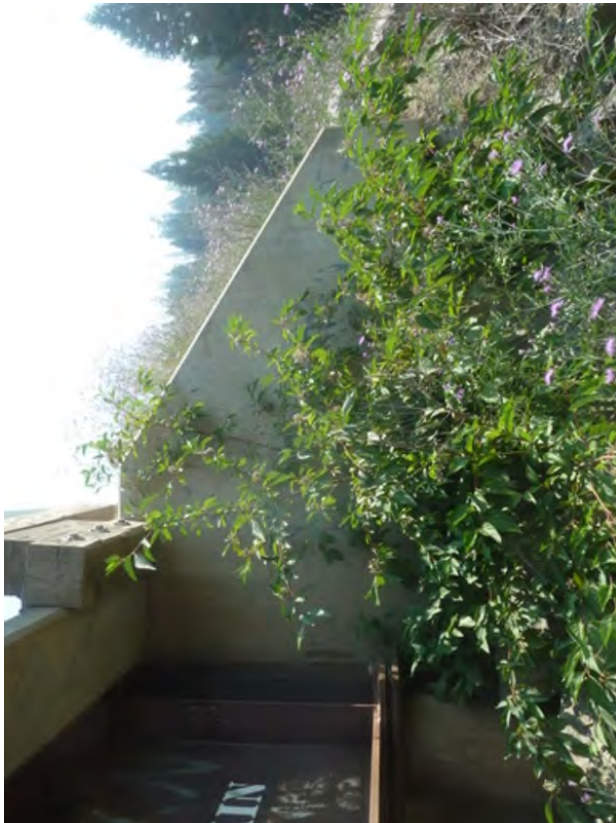
Figure 25: Right end upstream wingwall.
