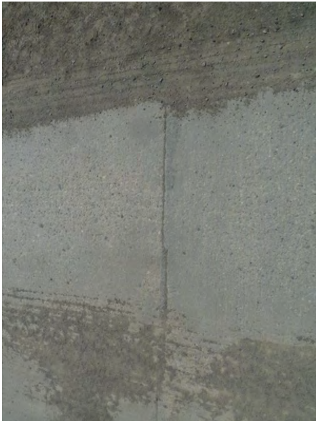
Figure 17: Typical grouted deck panel joint.
