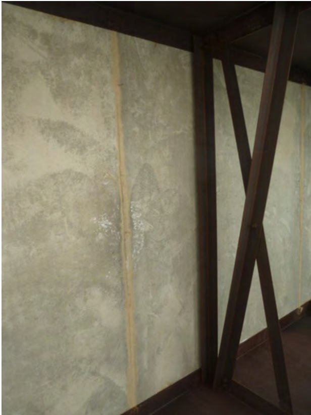
Figure 18: Typical underside of deck.
