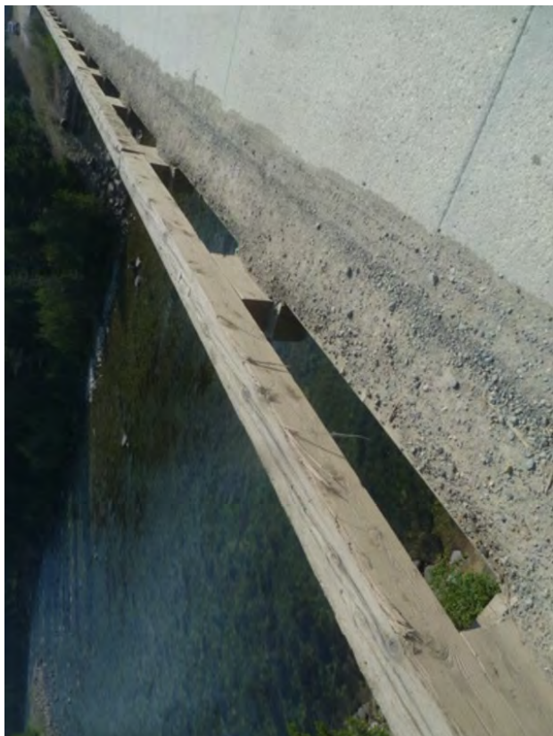
Figure 10: Typical condition of downstream curb.
