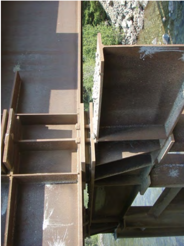
Figure 30: Span 1 bearing at Pier 1
